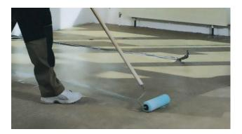
• Primer is used before self-leveling cement, to close the pore and crack on subfloor, reduce the absorptive character, at the same time, it can increase the adhesive ability between subfloor and adhesive.
